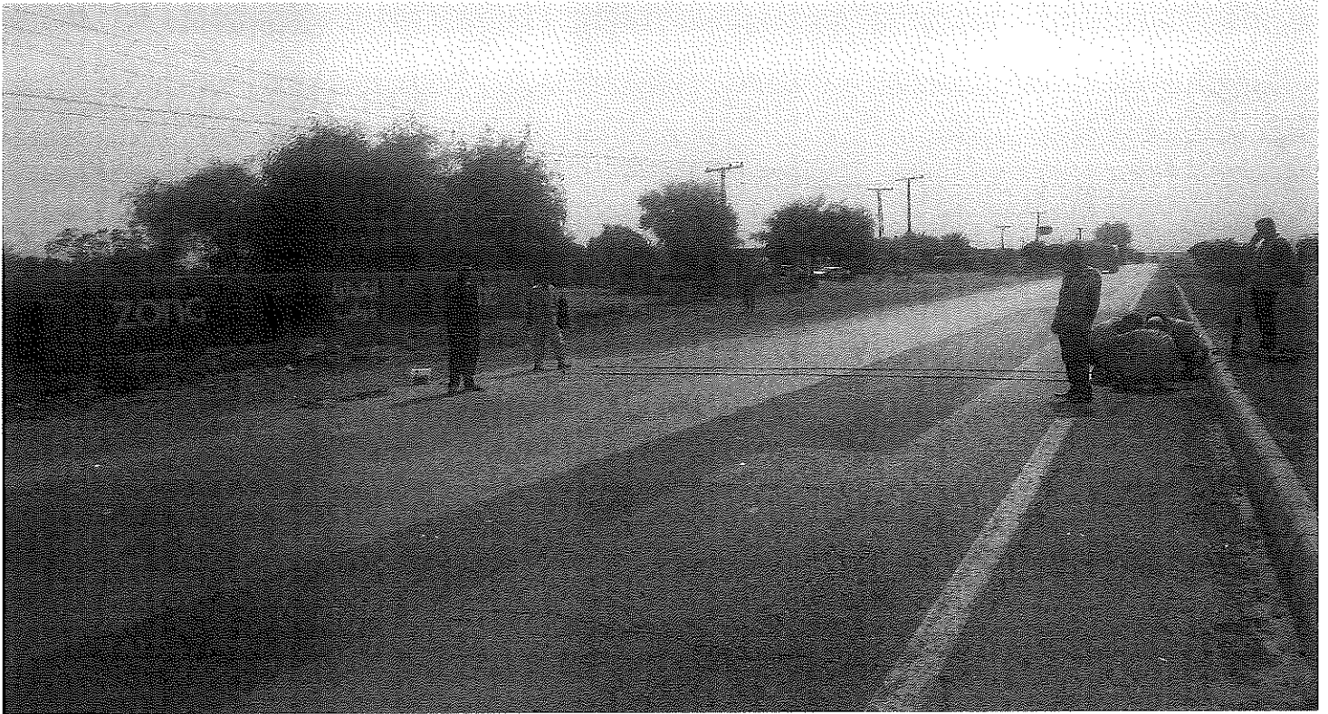
Engineer installing Metro Counter
